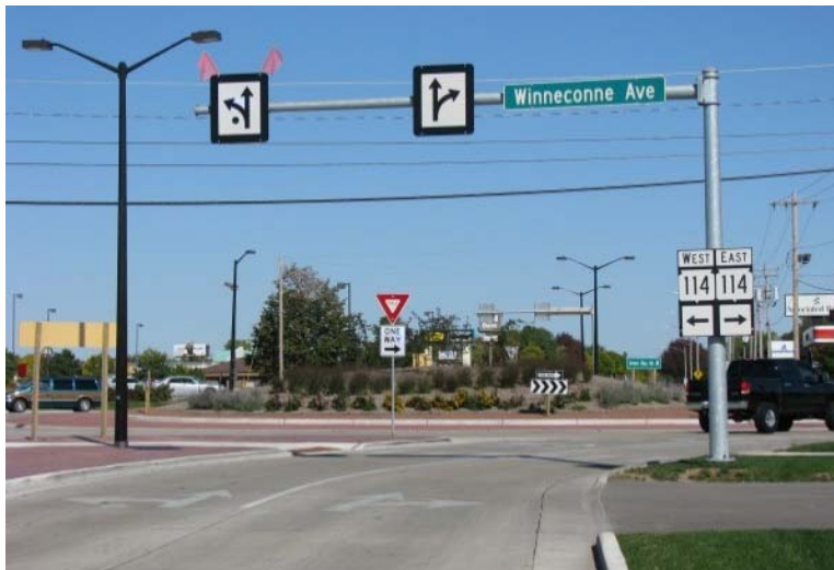
Figure 2. Overhead Lane Signs
